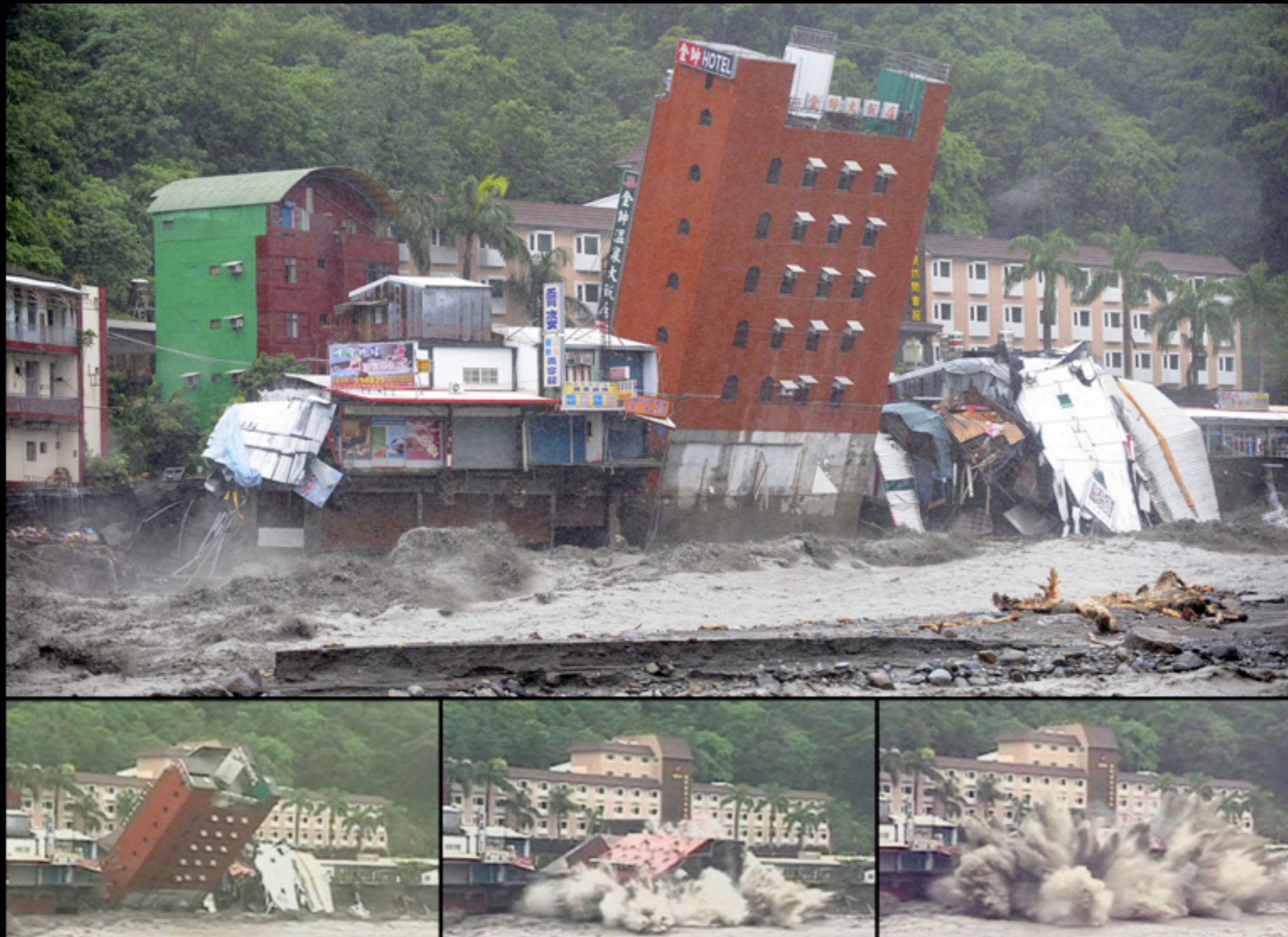
A hotel building leans before falling in a heavily flooded river after Typhoon Morakot hit Taitung county, Taiwan, Sunday, Aug. 9, 2009. The six-story hotel collapsed and plunged into the river Sunday morning after floodwaters eroded its base - all 300 people in the hotel had been evacuated and uninjured, officials said. (AP Photo / AP
